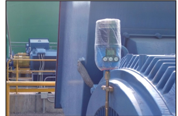
Automatic dispensers are safe, reliable, and easy to maintain delivering the exact amount of grease required.
