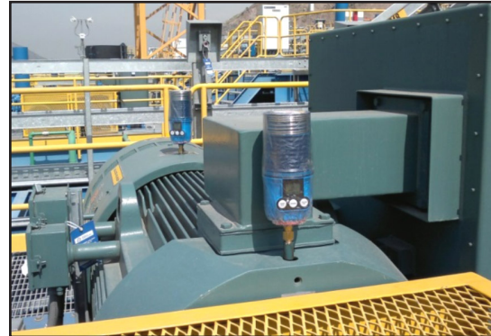
Chesterton electric motor reliability solutions installed.
